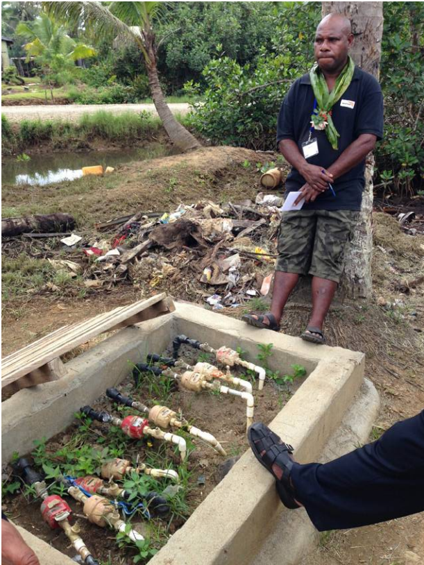
Informal communities in Suva can access mains water in Lami corridor, often with households sharing metered connections. Photo credit: Bronwyn Powell/CS WASH Fund Management Facility.
