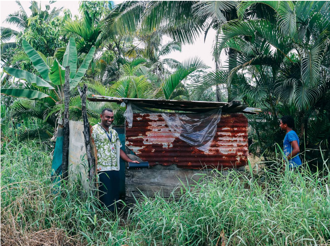
Maciu Nokelevu, Live and Learn Fiji, inspects a pit latrine in Lami corridor informal settlements. Photo credit: Fotofusion Fiji
